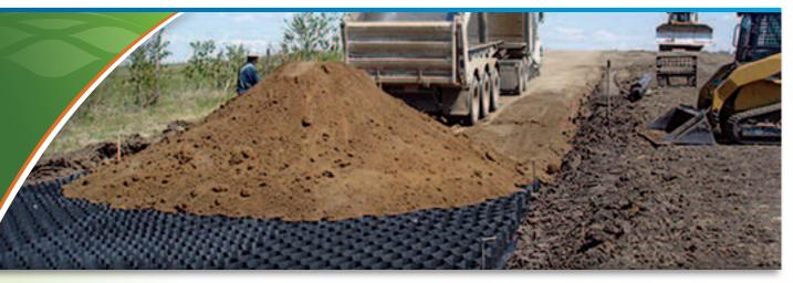
The GEOWEB® Load Support System is a proven, economical solution for challenging soil stability problems. The 3D structural system delivers benefits where soft soils are present, where inexpensive quality infill is unavailable or where traditional reinforcement methods are difficult to construct.
