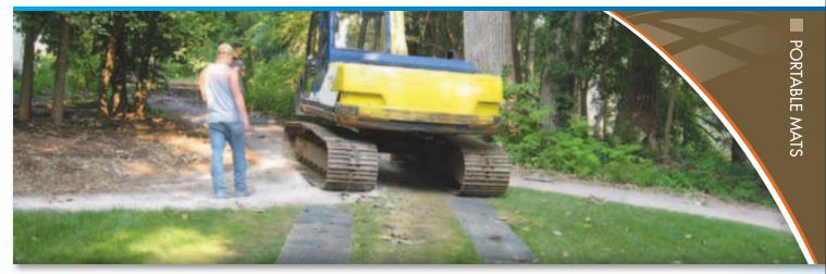
**GEORUNNER®** Surface Protection Mats are portable, economical and drivable construction mats. Their light weight (8 lbs.), easyto-handle size makes them ideally suited for transporting and deploying on construction sites.
