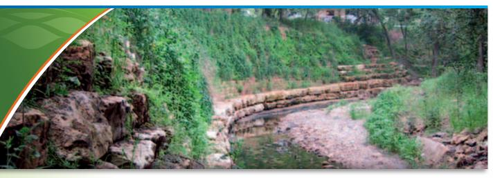
The **GEOWEB®** Channel Protection System stabilizes and protects channels exposed to erosive conditions of all types and can be designed with appropriate infill types to withstand even the highest velocities.
