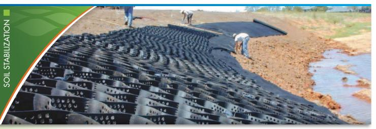
The **GEOWEB®** Shoreline Protection System stabilizes soils on shoreline embankments, creating a structurallystable environment for infill. The system minimizes erosion problems caused by water contact, surface flow and small scale wave action.
