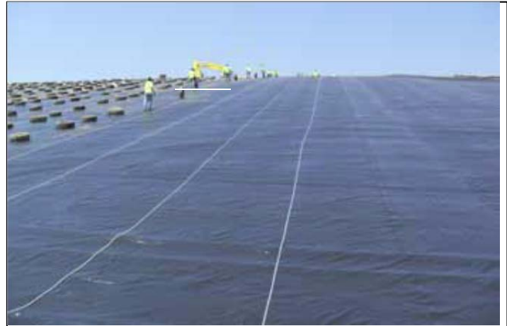
Temporary Rain Shed cover
